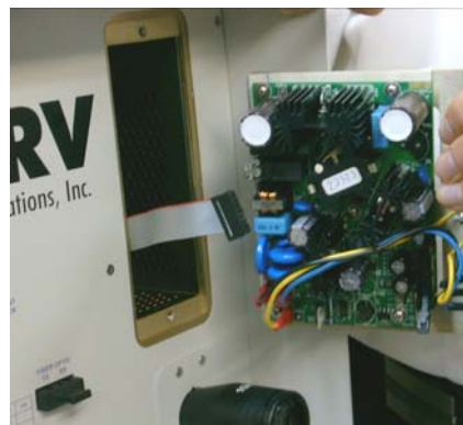
Figure I.3: Disconnected Flat Cable
