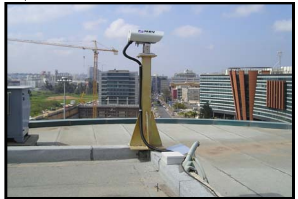
Figure 2.7: Floor Pedestal Mounting (using JMP and M015C)
