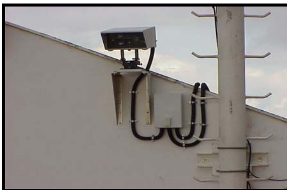
Figure 2.8: Wall Mounting (using JMP and JMB)
