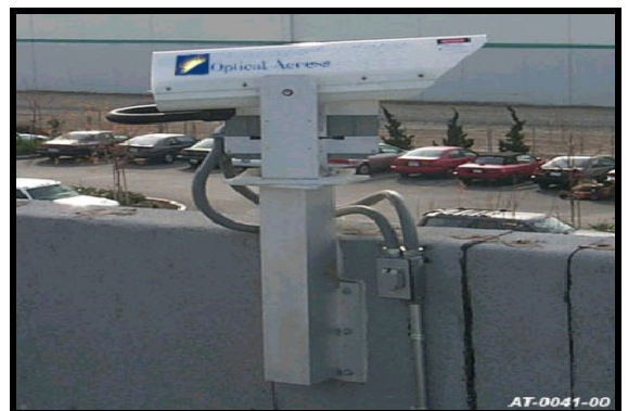
Figure 2.9: Wall Pedestal Mounting (using JMP and M054C)
