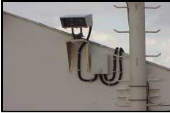
Figure 2.8: Wall Mounting (using JMP and JMB)
