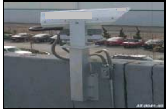
Figure 2.9: Wall Pedestal Mounting (using JMP and MO54C)
