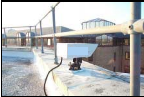
Figure 2.6: Parapet/Ledge Mounting (using JMP only)
