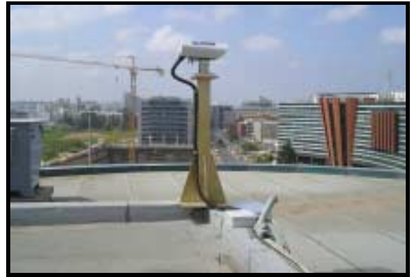
Figure 2.7: Floor Pedestal Mounting (using JMP and M015C)
