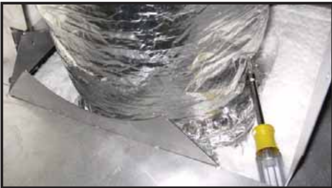
Figure 7.6. Install Insulated Flex.
