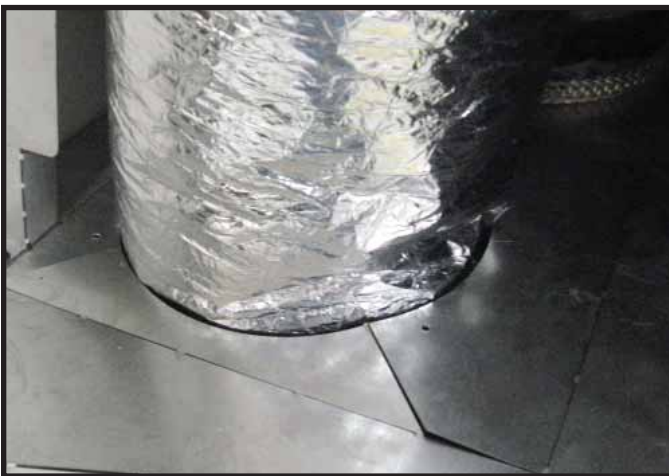
Figure 7.7. Bend Pre-cut Tabs Down.
