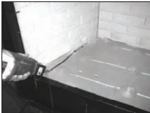
Figure 11.2. Using a saws-all, cut out the floor
