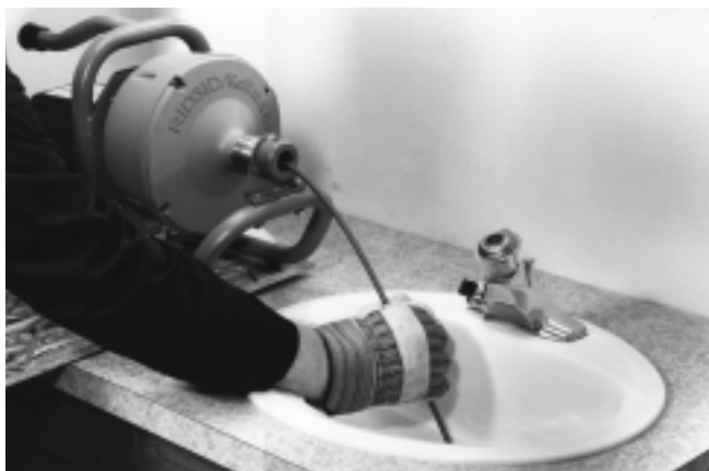
Figure 15 – Push cable down drain line keeping your control hand close to the drain opening
