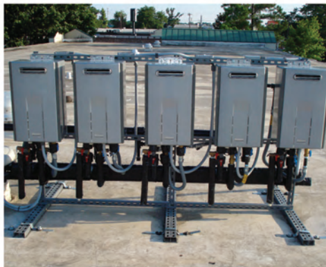
At this 40-room hotel, exterior units are mounted on the rooftop with no additional venting. Hotel owners have experienced 50 percent reduction in therms per occupant room.
