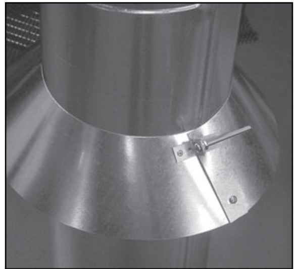
Figure 2.22 Assembling the Storm Collar Around the Pipe
