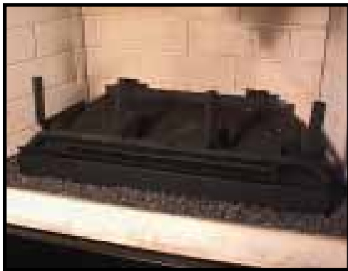
Figure 6 - Placing the Grate Assembly
