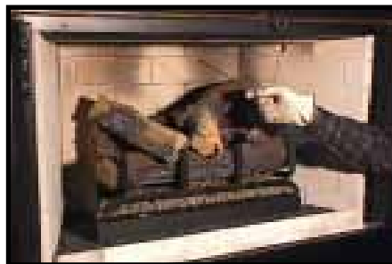
Figure 16 - Checking for Spillage
