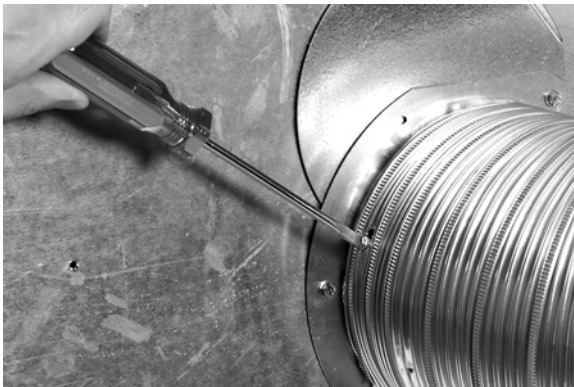
Fig. 13. Connecting Bypass Duct to Bypass Collar.
