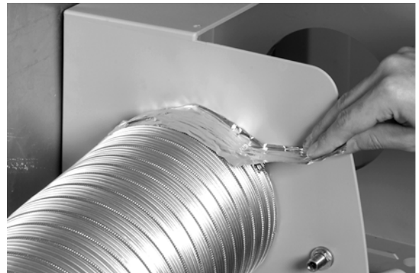
Fig. 15. Sealing connections with tape.
